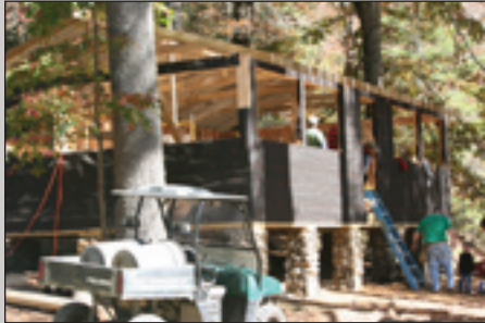
The new cabin of Avalon begins to take shape
